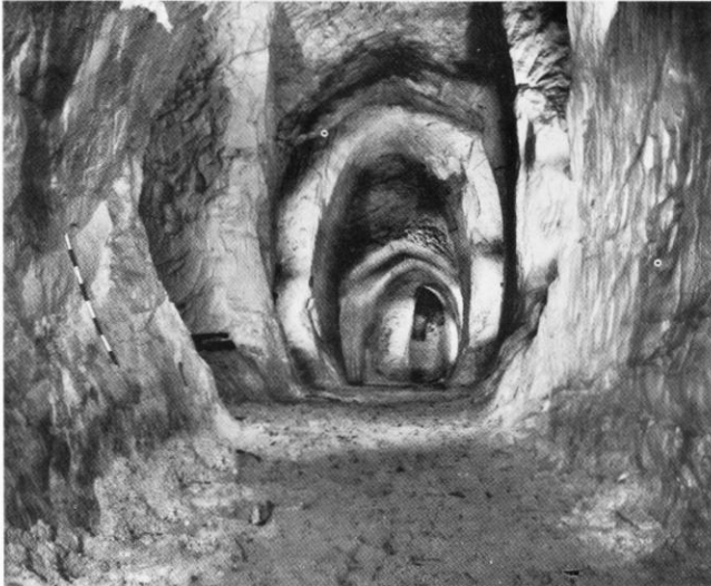
Reigate Lodge North mine: this impressively spacious mine tunnel (and the whole Reigate Lodge complex) is currently accessible only via a wide, deep vertical shaft which enters via the ceiling. At the far end only the right hand side of the gallery has been excavated. The scale bar is 21 inches.
